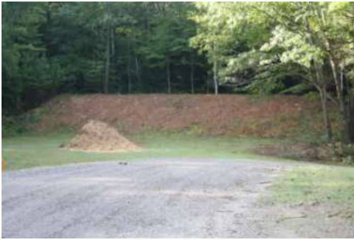
600 Yard Firing Point Rehab.
